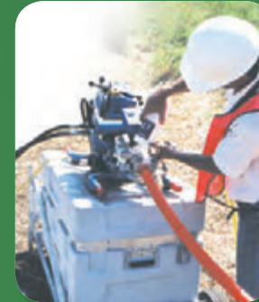
Fiber Optic Cable Blowing Method Pages 134-135
